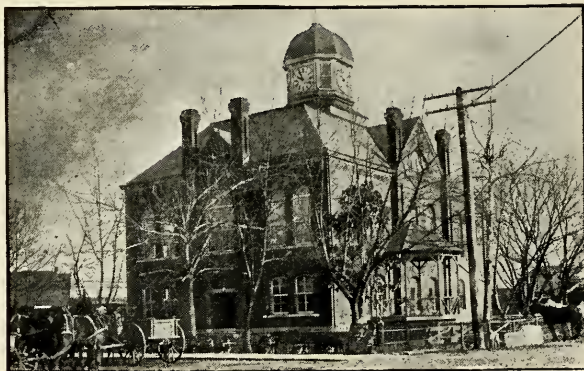
COURT HOUSE, KENNETT
